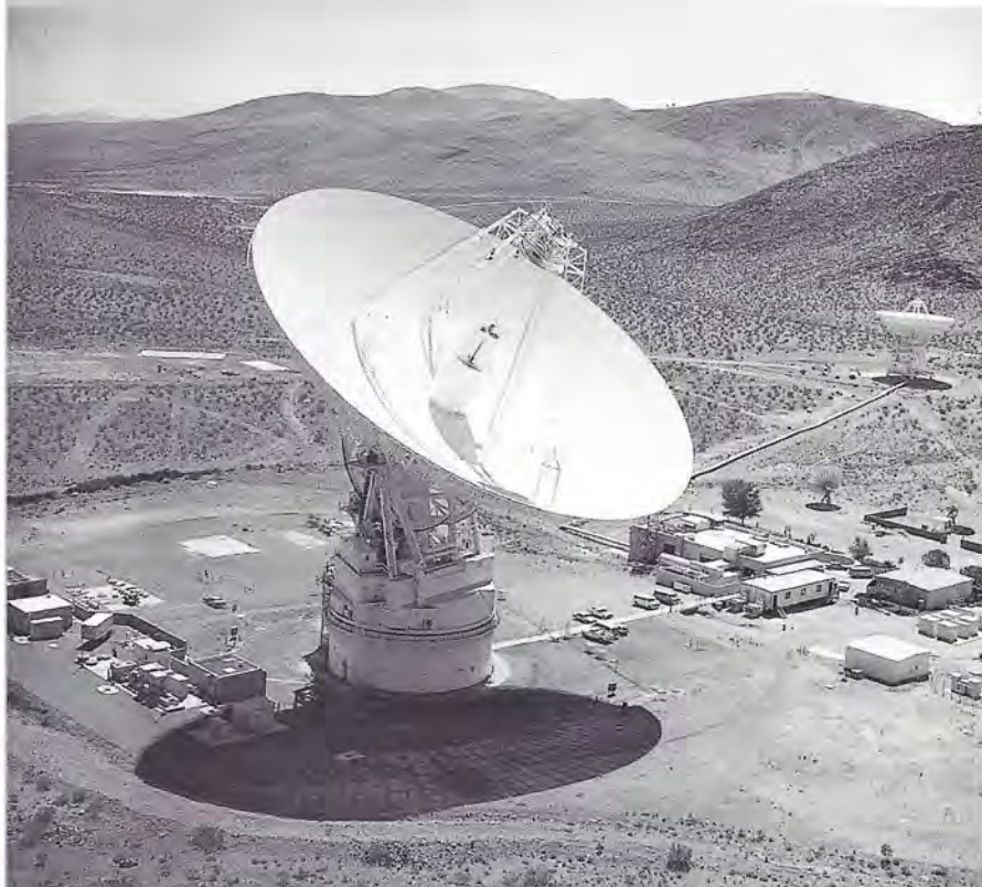
The 70-meter Deep Space Station (DSS) at the Goldstone Deep Space Communications Complex in California dominates this image. The 34-meter high-efficiency DSS can be seen off to the right. The building between them houses the signal processing center for the complex. The 70-meter DSS has three feedhorns, each leading to a different configuration of equipment. Operators select a feedhorn by repositioning the subreflector, poised above the dish on four legs. Goldstone's desert location helps minimize radio noise.
