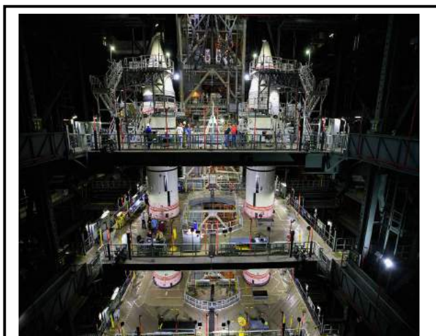
Stacking is complete for the twin Space Launch System solid rocket boosters for Artemis I mission. Over several weeks, workers used one of five massive cranes to place 10 booster segments and nose assemblies on the mobile launcher inside the Vehicle Assembly Building at NASA's Kennedy Space Center.
