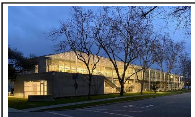
The recently completed Biosciences Collaborative Facility at the Ames Research Center (pictured above) is a ~40,000 square-foot laboratory that enables cutting-edge biology research.
