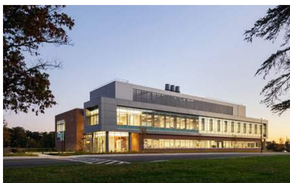
NASA's Instrument Development Facility at Goddard Space Flight Center (pictured above) is a new, Leadership in Energy and Environmental Design (LEED) certified, 54,000 square-foot facility and home to the Planetary Environments Laboratory operations, a cornerstone for the continued search for evidence of life on other planets.
